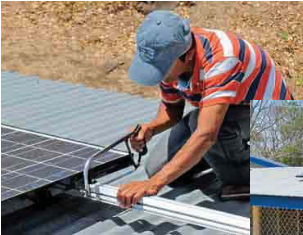
Above: A Las Cuchillas community volunteer cuts the EZ mount rack for the battery-based PV system.
